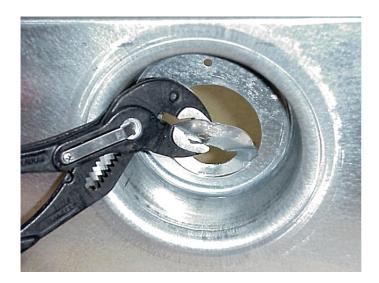
Detach the pre-drilled adaptation plate from the drain sleeve.
