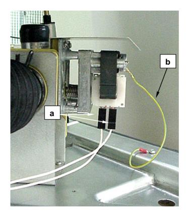
Connect electrical supply wiring (a) and ground wire (b).
